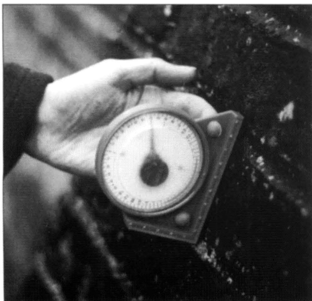
Fig. 5. Measuring the reclamation of a wall using a purchased 'level angle finder'.
