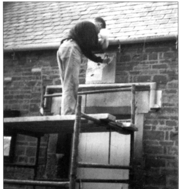
NE sundial being restored
